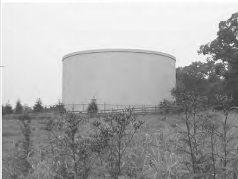
2.0 MG water storage tank in Sellersburg, IN for the Silver Creek Water Corp. Engineering by Jacobi, Toombs & Lanz, Inc.
